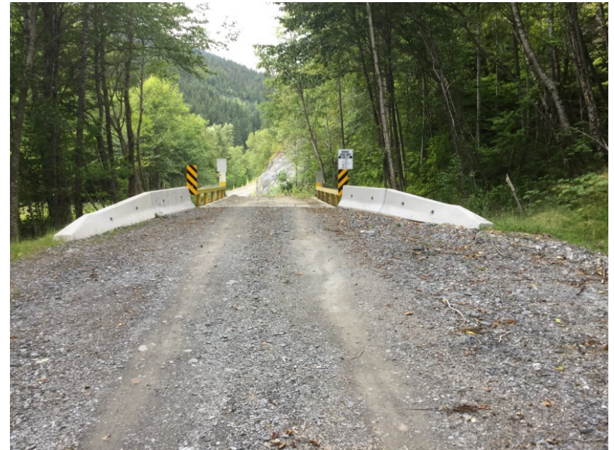
Left Approach Facing Bridge
