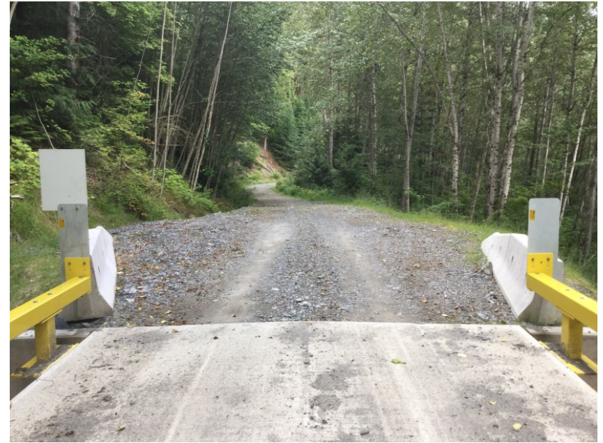
Left Approach Facing Away From Bridge
