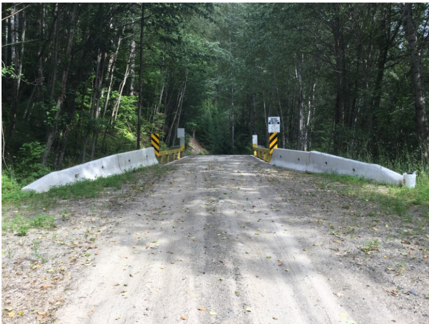
Right Approach Facing Bridge
