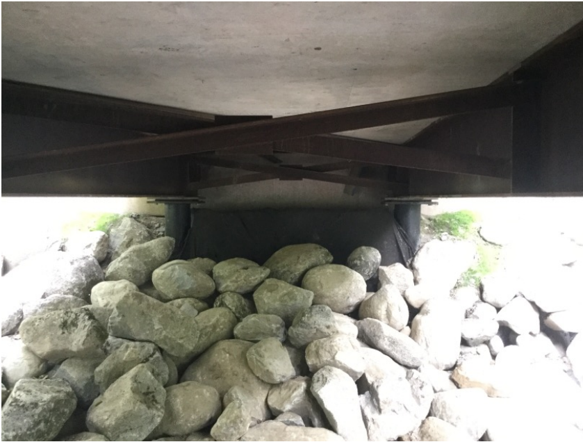
Left Bank Abutment
