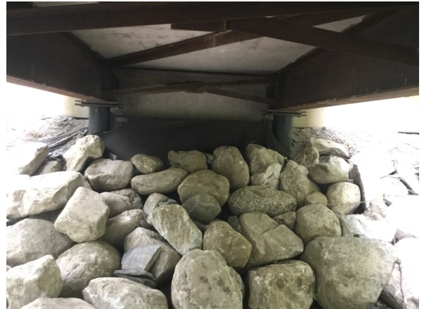
Right Bank Abutment
