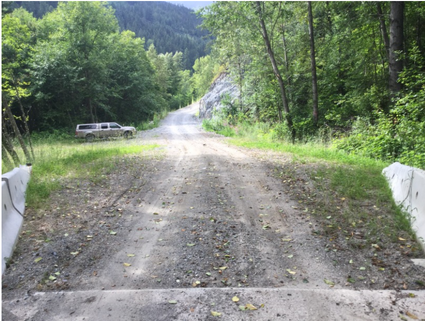
Right Approach Facing Away From Bridge
